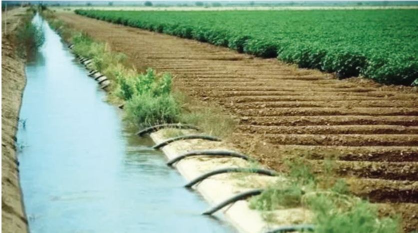
Fig 11c, Canal Irrigation System
